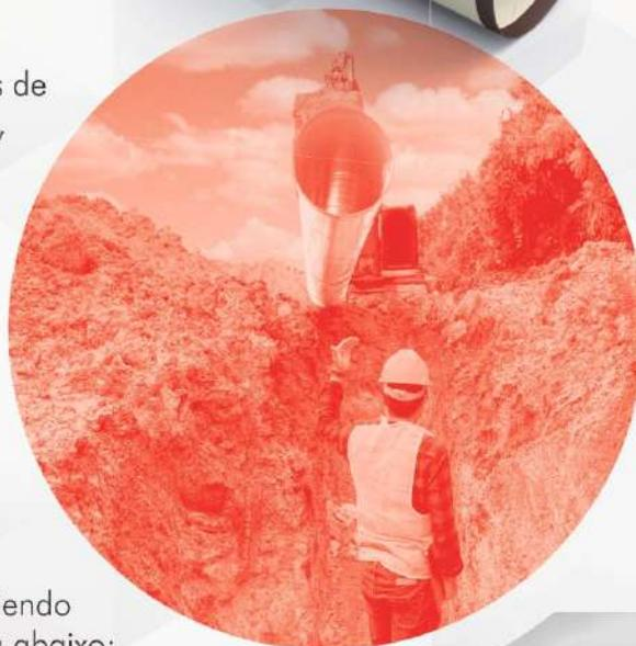
Tubos de Aço ASTM A1018 Gr. 36 - Norme AWWA C200
